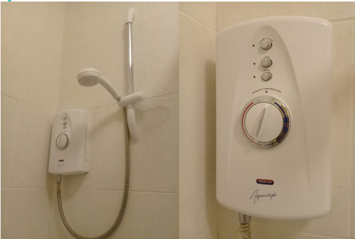
The wall unit in which the water is heated.
