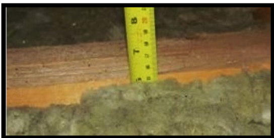
Figure 6.1: Measuring roof insulation thickness
