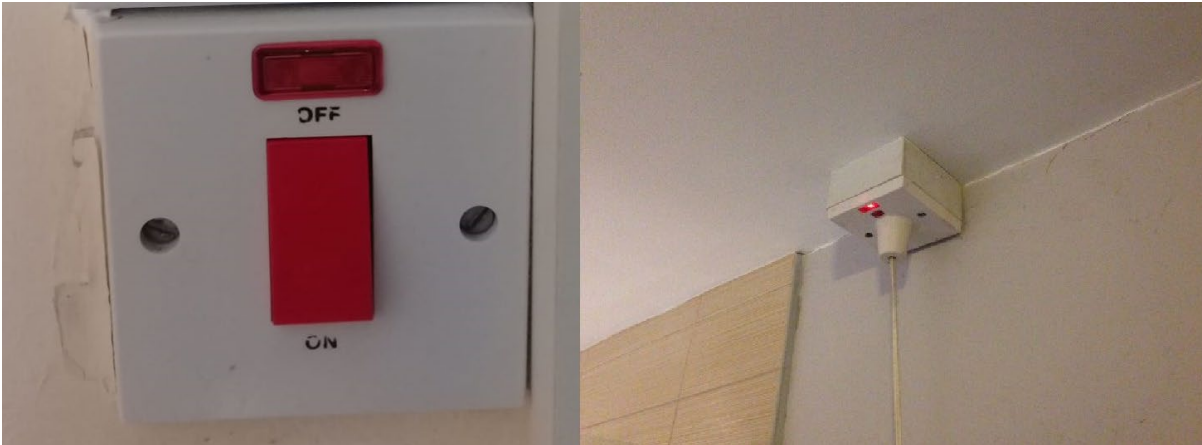
Figure 8.10 – A wall-mounted isolator switch (left), and a ceiling-mounted isolator switch (right) for an electric shower.
