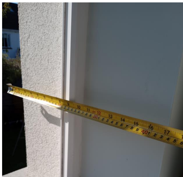
Figure 4 – Wall thickness as a verification indicator
