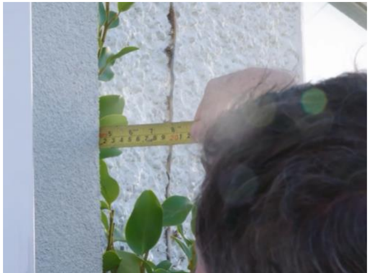
Figure 7 - EWI upgrade evidence at boundary wall
