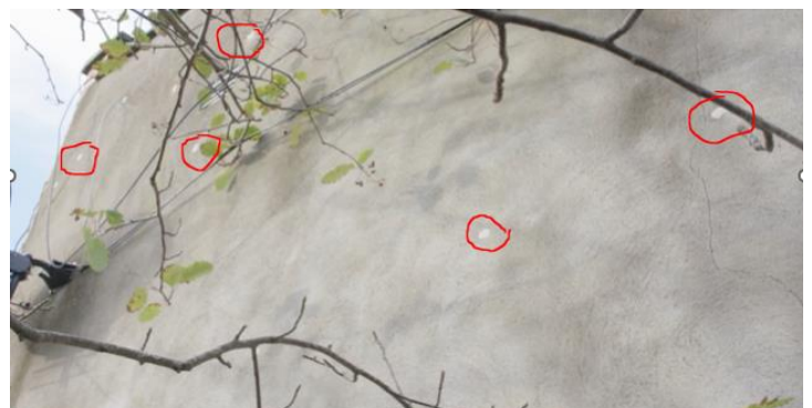
Figure 9 - Drill pattern example for CWI upgrades
