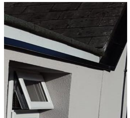
Figure 5 - Metal flashing at soffit level
