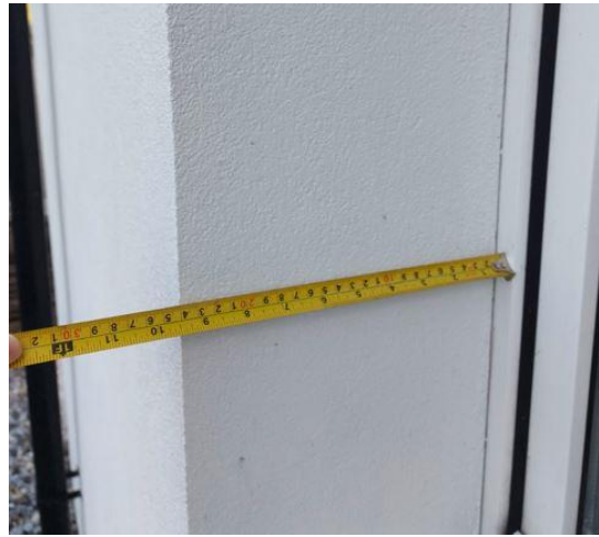
Figure 3 – Larger exterior reveal depth (240mm)
