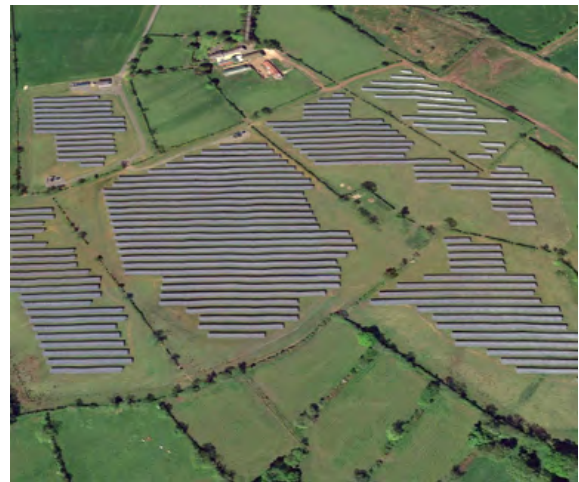
4.8MW Solar Farm
