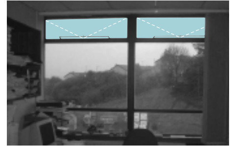
Location of the openable window section of the windows in the new part of the building.
