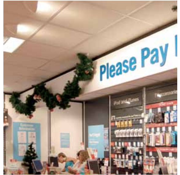
Fig.1 'Accent' lighting using 70W metal halide lamps
