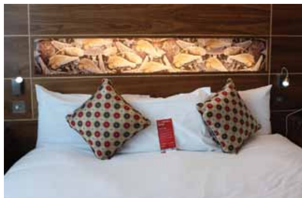
Fig.6 Concealed T8 high efficiency tubular fluorescent and LED reading lights
