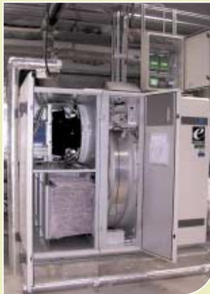
An internal view of the new AHU, including extract air fan, thermal wheel, air inlet filters, and cyclon control panel
