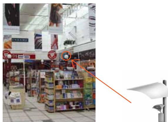
Fig. 6 Convert ineffective globe light to uplighter with integrated reflector
