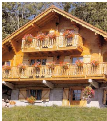
Wood chalet with geosolar heat pump in the Drôme region, France.
