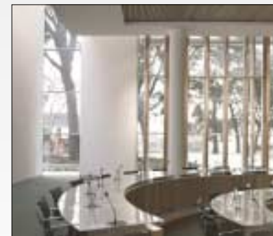
In the Council chamber, concealed roof lights reflect day light off the back wall to provide glare free daylight.
