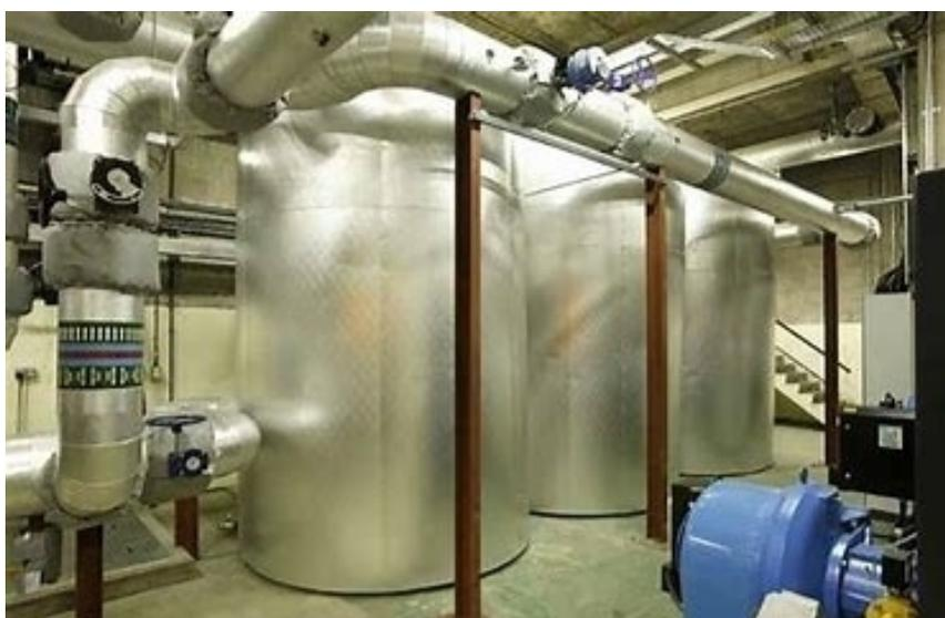
Using thermal storage changes the operational demands on biomass boilers and any back-up fossil-fuel boilers, changing the design economics of a biomass system. This is because thermal stores enable smaller biomass boilers to operate continuously for longer periods than larger boilers that must vary output significantly or even start-up and shutdown frequently. This means improved efficiency and use of the biomass boiler. A smaller biomass boiler will also be cheaper.
