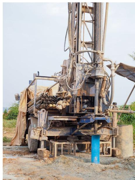
Figure 14: Water well being drilled
