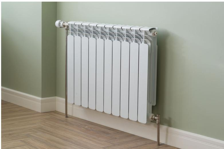
Figure 10: Low-temperature radiator
