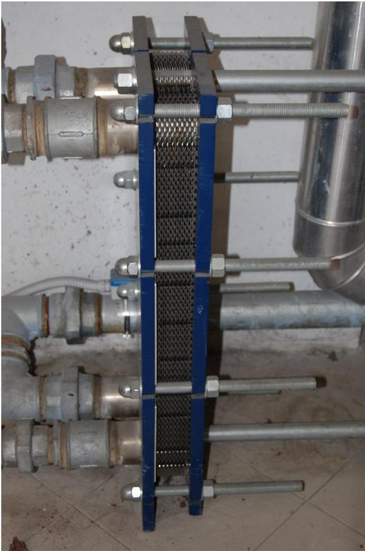
There are many types of heat exchanger, but most systems will use plate heat exchangers (see Figure 10) or plastic heat exchangers. Plate heat exchangers are considerably more compact and can be located in plant rooms where they can be serviced easily. However, they use very small capillaries in the heat exchanger that are prone to blocking because of debris or fouling by dissolved minerals (e.g. iron).
