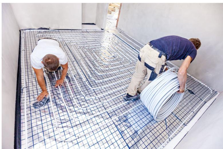
Wet (also known as hydronic) underfloor heating involves laying loops of plastic pipes (usually between 10 mm and 20 mm outside diameter) through which water is pumped. The pipes are either located inside a concrete floor or in grooved aluminium plates within a floor screed. The pipes are arranged in loops connected back to manifolds. A room can have one or more loops controlled by a thermostat.
