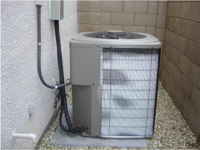
The design of the condensate drainage system must take account of the fact that the condensate can freeze due to cold air from the heat pump itself. You should allow adequate space around the heat pump to avoid the development of a 'cold well' (localised area of very low temperature), which can exacerbate this effect.
