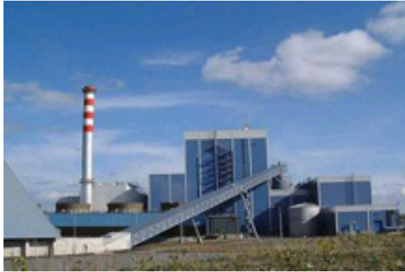
Figure 11: Power station (Edenderry Power Plant, Bord na Móna)
