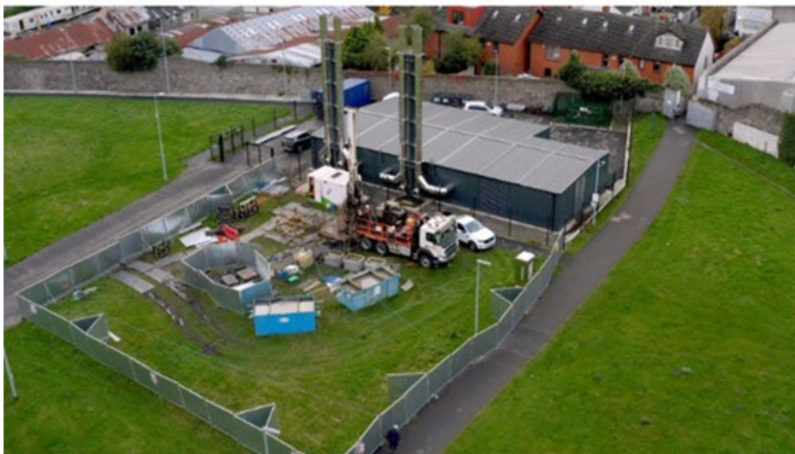
Figure 34. Borehole at TUD
