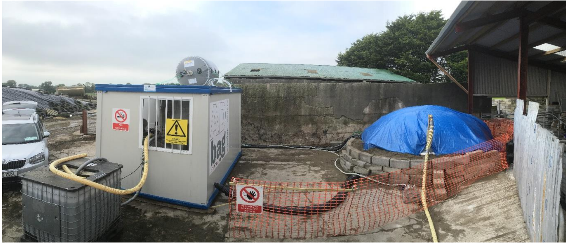
Fig. 13 - Final set up of the pilot plant at Hayes Farm, Two Mile Borris, Co, Tipperary.
