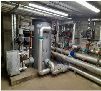
1,000 litre Buffer Tanks and Heat Exchanger
