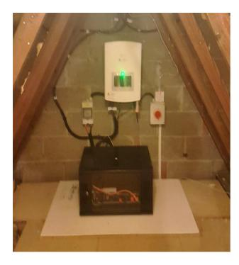
Battery is installed in a suitable enclosure fixed in place on a fire-resistant surface or substrate (Class o) which extends 150mm beyond the edge of the system.
