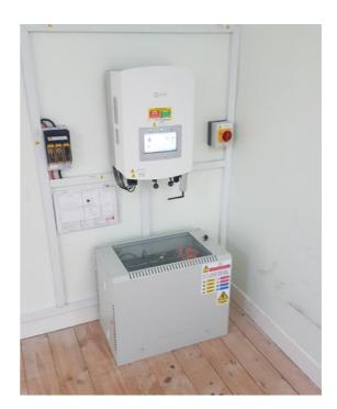
Battery is installed on a combustible material and is not fixed in place.
