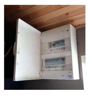
No Dual supply warning label on fuseboard. Inadequate labelling may create a safety issue for the homeowner or future installers.
