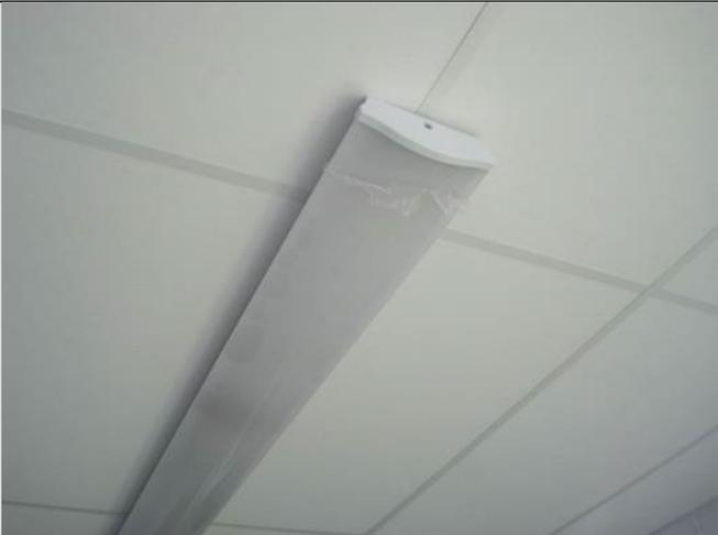
LED in new fittings are integral to fittings rather than a removable part. The light fitting shown above is an LED.
