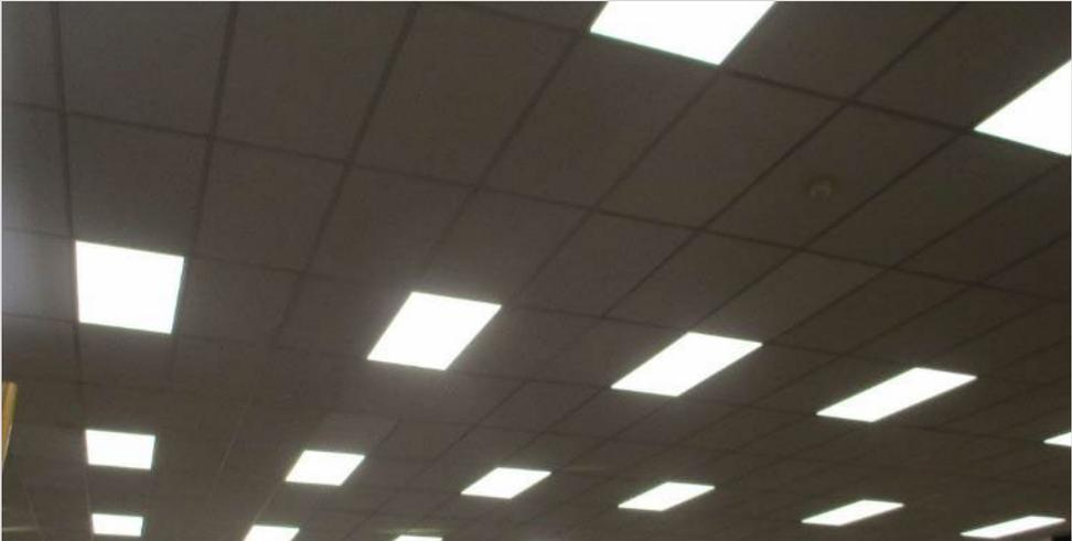
LED panels have replaced recessed T-8 fittings in this shop.
