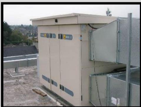
The multi-split outdoor unit is as follows. There are four units, each serving a number of indoor units. In this example, they can both heat and cool the building.
