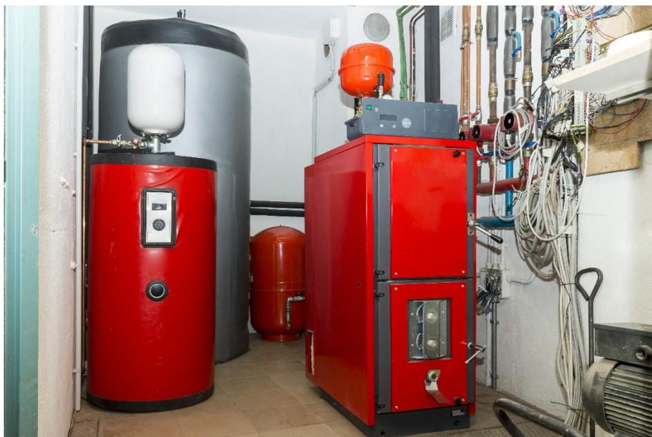
Figure 3.2: Plant room with small biomass boiler and thermal store
