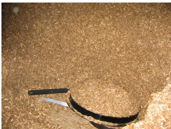
The type of storage will largely dictate the type of delivery vehicle. Compatibility with potential suppliers' vehicles should be thoroughly checked. Normally wood pellets are delivered by lorry with a blower system. Wood chips are often delivered by a tractor with tipper trailer, a large lorry with tipper, or via walking floor fuel delivery system.
