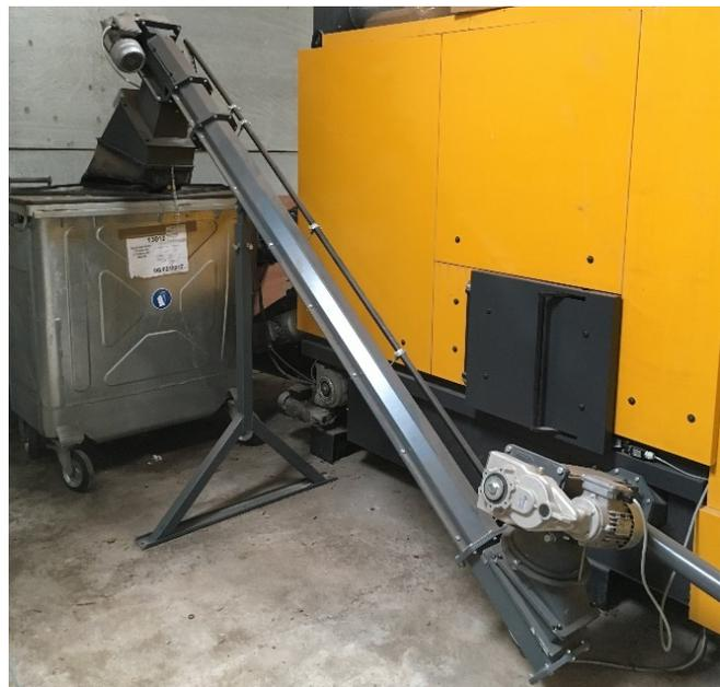
Figure 6.1: Conveying ash to a separate container within the boiler house
