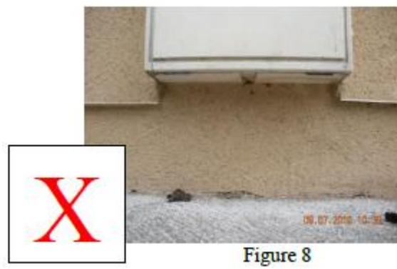
The above Figures 7 and 8 show the surface mounted meter box with the external insulation having been installed to cover both the gas installation inlet/outlet pipework and a large amount of the meter box.
