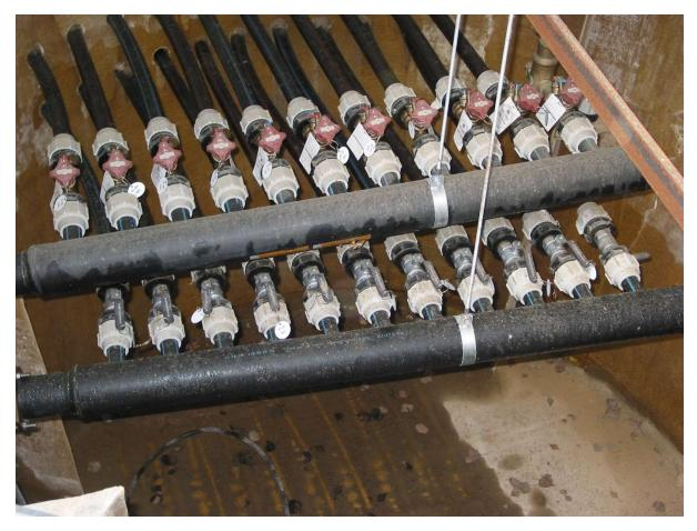
Manifold chamber for a large lake collector with valves and flow regulators.
