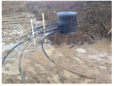
Manifold chamber with lid prior to back-filling
