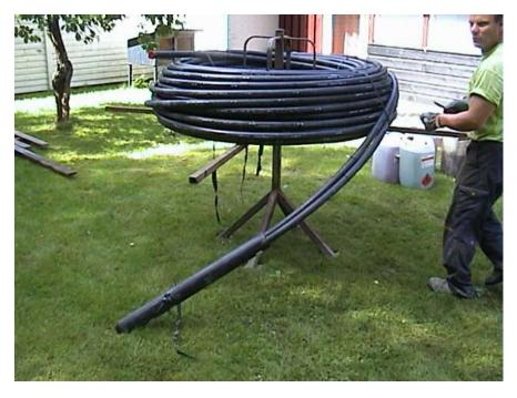
Borehole probe on a turntable to allow unwinding and insertion to the well whilst filled with water.
