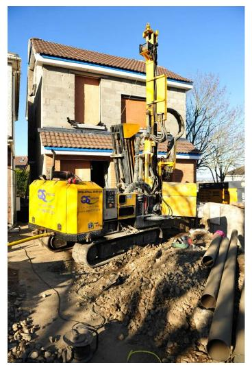
Mini Drilling rig making a borehole in a suburban Dublin house- with a tiny garden, the owner elected to use a borehole as the more aesthetic solution over an air to water heat pump.
