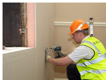
3. Internal Wall Insulation
