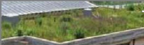
GREEN ROOFS help mitigate against URBAN HEAT ISLAND EFFECT by increasing the building's solar reflectance index and delaying surface water run-off
