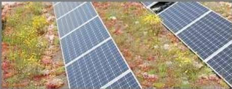
1.5 PV PANELS per apartment provide energy efficient fuel for apartments and achieve renewable energy compliance with Part L requirements for DEAP analysis
