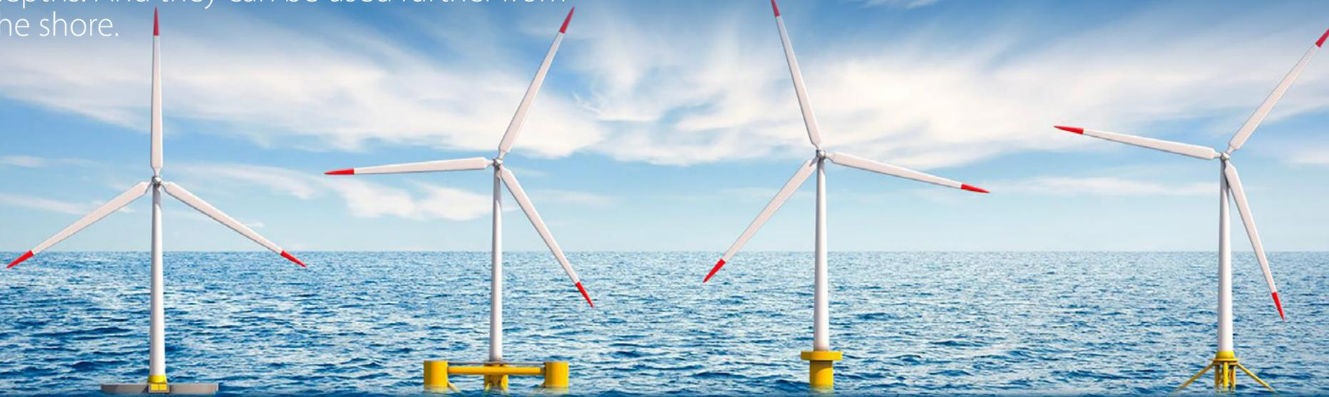
There are differing floating offshore wind designs that need to be tested at full scale, here are some examples.
