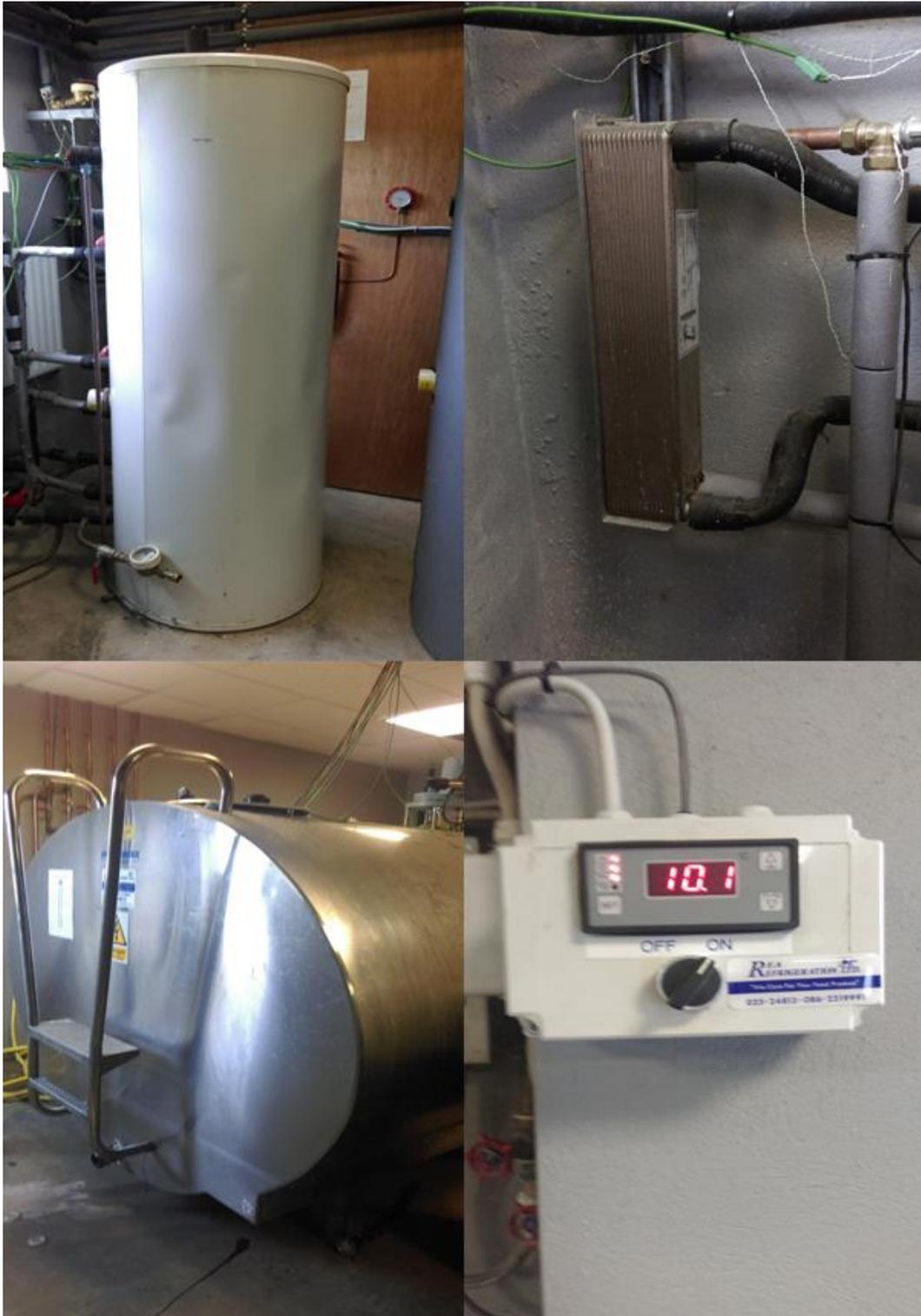
Figure 8: Equipment for heat recovery experiments. Clockwise from top left: 500L water tank heated using heat from Direct Expansion (DX) cooling tank; Heat exchanger to transfer waste heat to water; Temperature sensor control for DX tank; DX tank.
