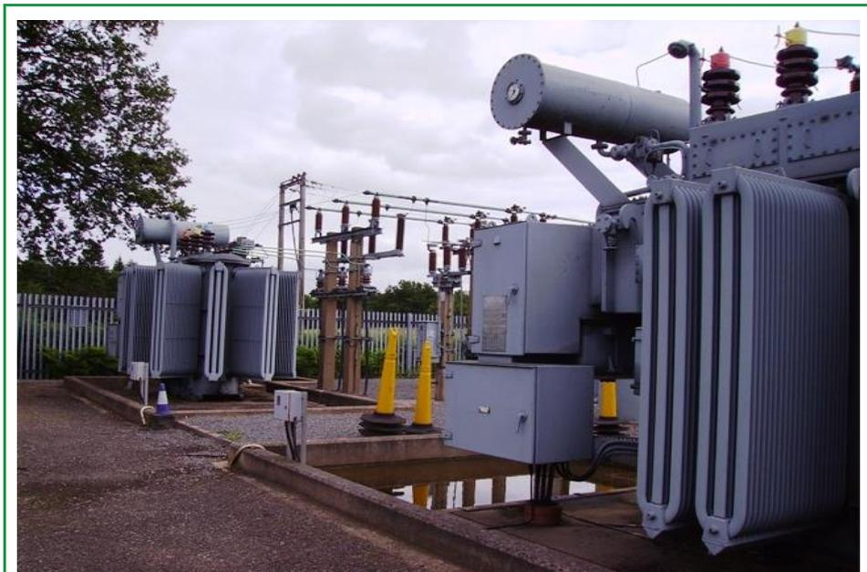
**FIGURE 19 – A TYPICAL TWO TRANSFORMER PRIMARY SUBSTATION**
