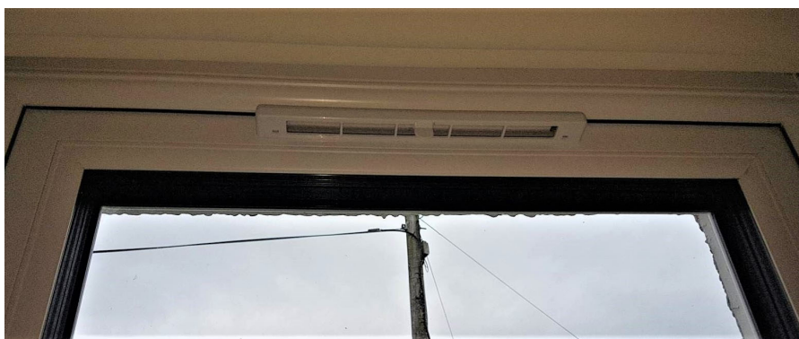
Figure 4: Background ventilation – window ventilator (adjustable)
