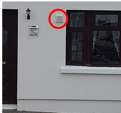
Figure 3: Permanent ventilation – outdoor view
