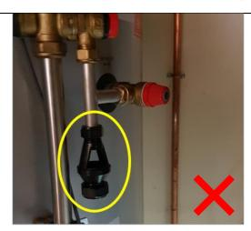
Figure 7: Incomplete Installation
