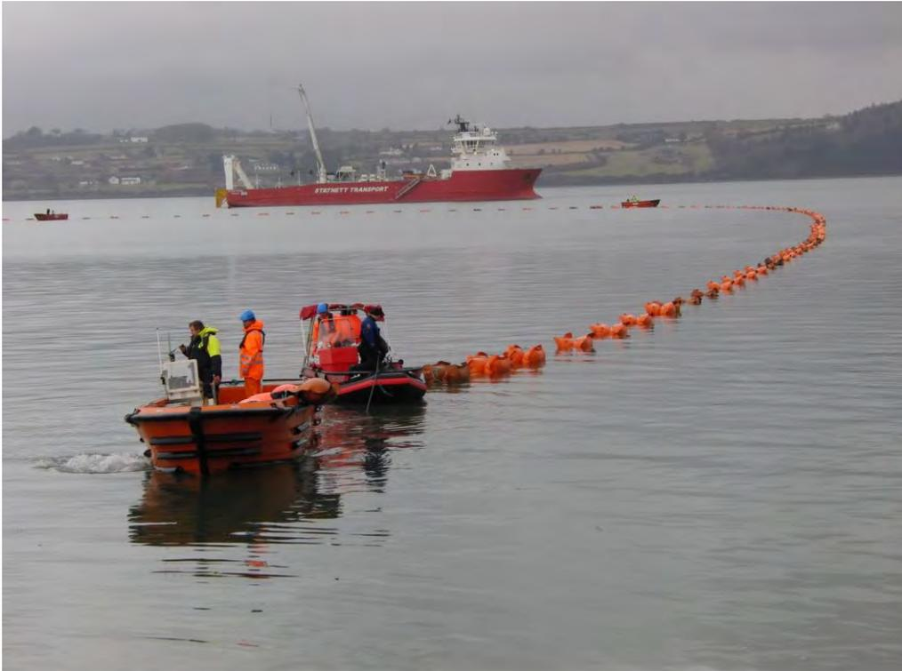
Figure 4-23: Shallow water cable deployment
