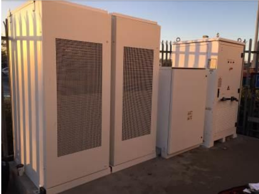
Figure 8. Completed Tesla Powerpack System
