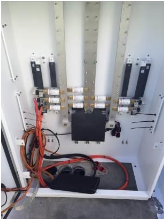
Figure 7. DC Link Box Internals
