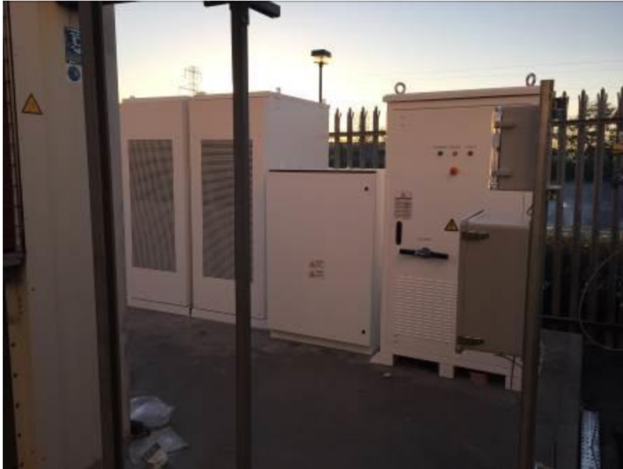
Figure 10. Completed Tesla Powerpack System
