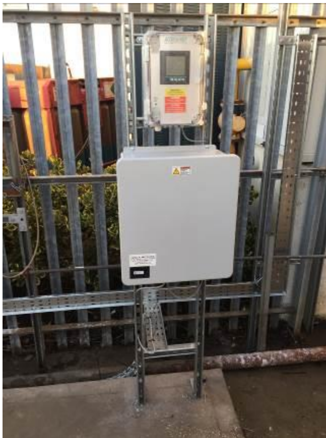
Figure 9. Master Controller and Metering
