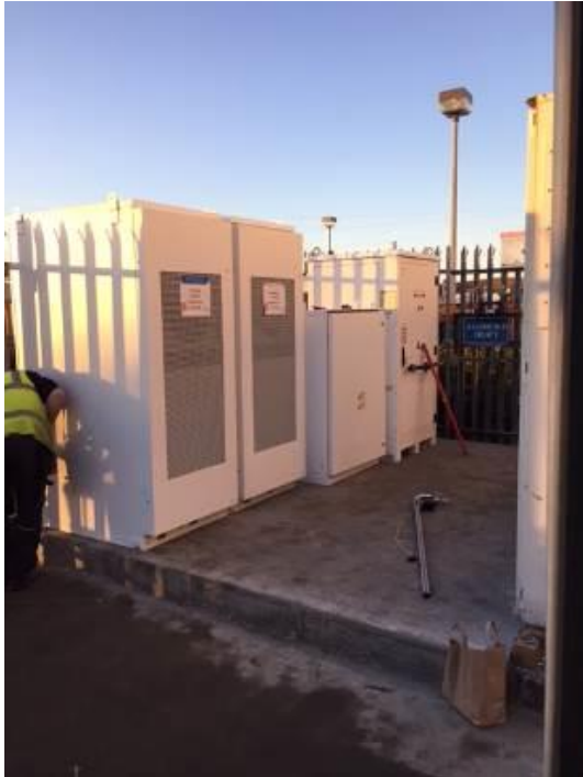
Figure 6. Installed major components on concrete foundation
