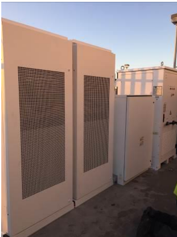
Figure 11. Completed Tesla Powerpack System
