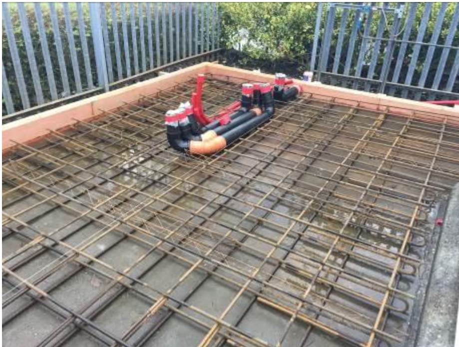
Figure 4. Foundation pad during installation before concrete pour
