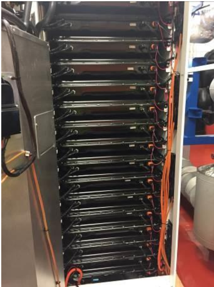
Figure 5. Internal components of 100kWh/50kW Powerpack – 2 of these installed at Boston Scientific
