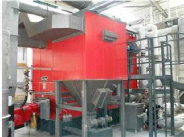
**Figure 10: Example Biomass boiler: Binder biomass boiler (from the 500 kW-10 MW range)<sup>17</sup>.**
