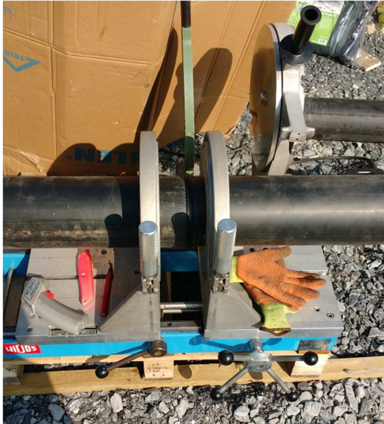
Figure 10: Butt Welding of GeoKOAX sections.
