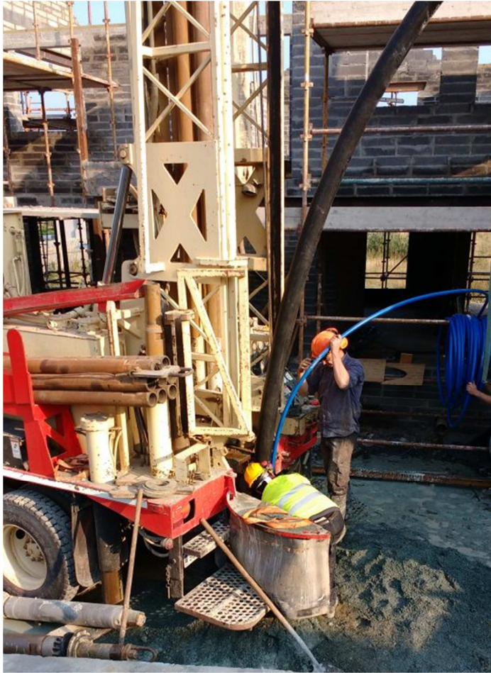
Figure 11: Installation of the welded of the GeoKOAX collector down the borehole with grout tube.
