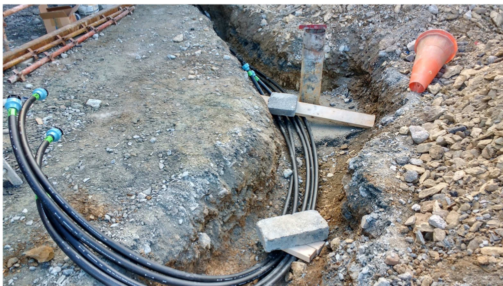
Figure 13: Trench work, flow/return pipes and cased borehole.
