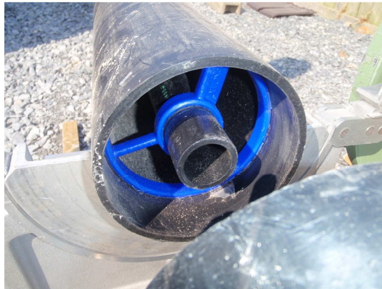
Figure 2: View of the inner and outer tubes of the GeoKoax during welding.
