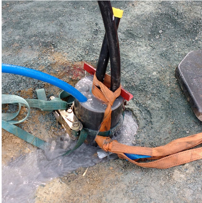
Figure 12: Grout entering via blue pipe, and displacing water out the top of hole.
