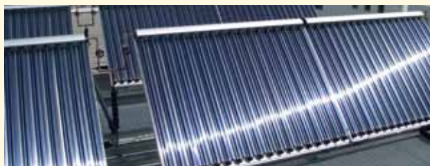
A LATENTO installation on the roof of the Playmobil Funpark on Malta
