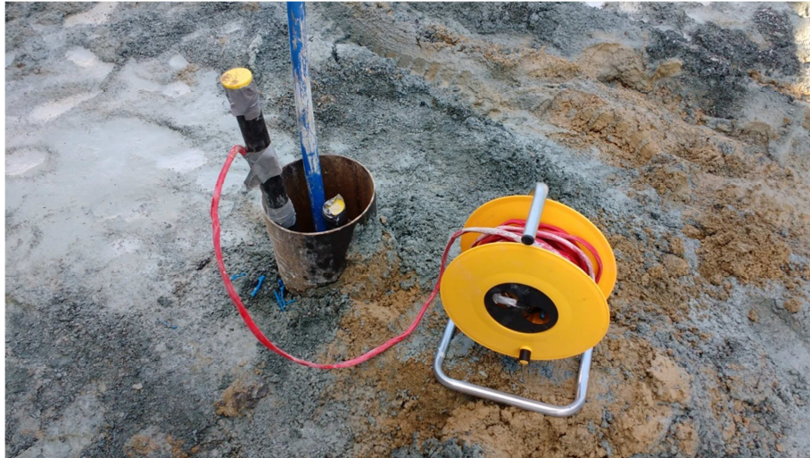
Figure 15: 4 thermocouples cables (in red wrap) inserted into the GeoKOAX borehole.
