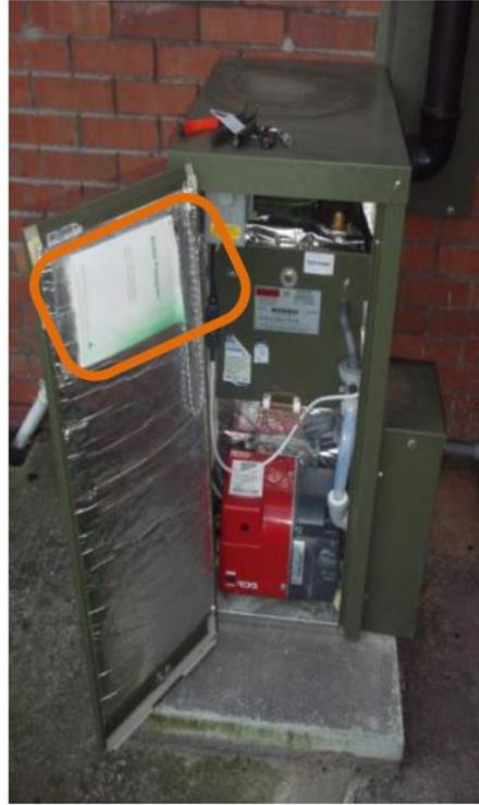
For the oil boiler above, the log book is in a sleeve attached to the inside of the front section of the boiler. It has a retainer (chain) so as it can't be removed from the appliance.
