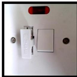
Boiler manuals give details of the fuse sizing. A 5-amp fuse must be installed for oil fired systems. Higher fuse ratings can be unsafe and will fail an inspection. A 3-amp fuse must be used for gas-fired systems.
