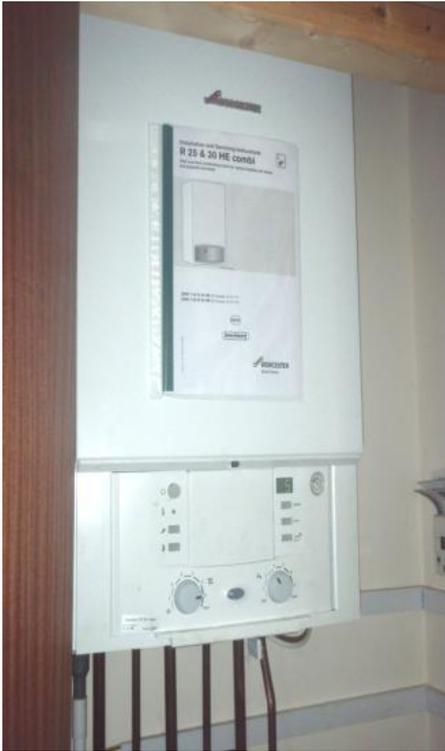
On the above gas boiler, the log book is placed inside a transparent plastic holder and securely fixed to the front of the boiler. This could also be placed on the inside door of any boiler enclosure if preferred by the homeowner.
