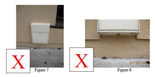
The above Figures 7 and 8 show the surface mounted meter box with the external insulation having been installed to cover both the gas installation inlet/outlet pipework and a large amount of the meter box.
