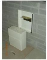
Figure 2a, 2b, Surface Mounted Meter Box [1]
