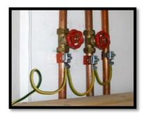
Older houses often have bonding wires of 6mm<sup>2</sup>, 4mm<sup>2</sup>, 2 mm<sup>2</sup> or even no bonding at all.
