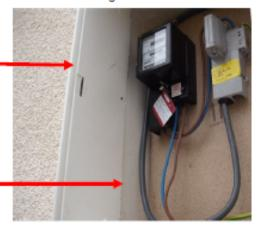
Meter cabinets are manufactured to a specific standard to give protection in the event of fire. Do not use alternative materials to modify the meter cabinet.
