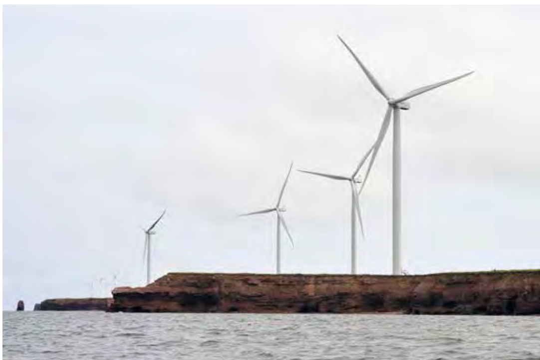
Figure 3. Wind Energy Institute of Canada (WEICan) R&D Wind Farm 2-MW DeWind D9.2 wind turbines (Photo credit: WEICan)
