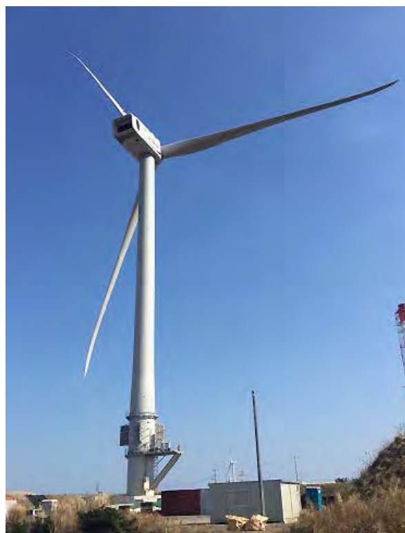
Figure 3. Hitachi 5-MW wind turbine HTW5.0-126 in Kamisu (Source: Hitachi, Ltd.)
