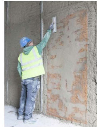
Figures 52 and 53: Insulating cork lime plaster sprayed on an uneven wall with reinforcement mesh applied below finish coat (Photographs by Con Brogan for OPW)
