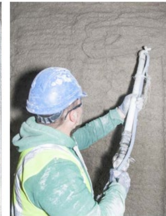
Figures 52 and 53: Insulating cork lime plaster sprayed on an uneven wall with reinforcement mesh applied below finish coat (Photographs by Con Brogan for OPW)
