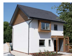
Figure 7: The Renewable House on the Innovation Park at BRE near Watford, Herts, constructed with hemp lime walls (Courtesy of Lime Technology)
