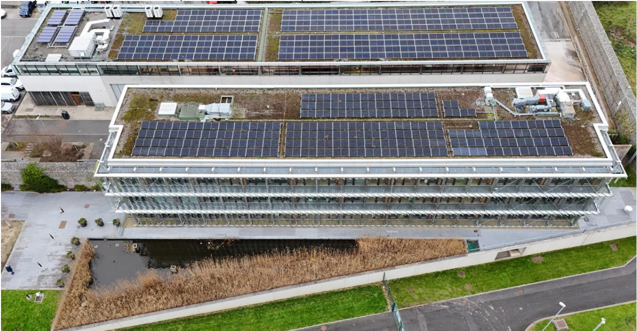
Finished Installation: Heat Pump and Solar P/V Array, Ballyogan Operations Centre
