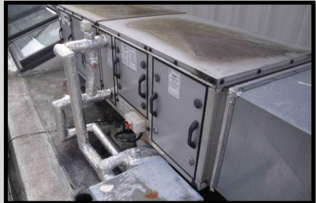
The Building Management System (BMS) image for this system is as follows. The remote extract section (shown at the top of the BMS image, but not in the photograph above) has no connection to the supply section, thereby demonstrating there is no heat recovery in this installation.
