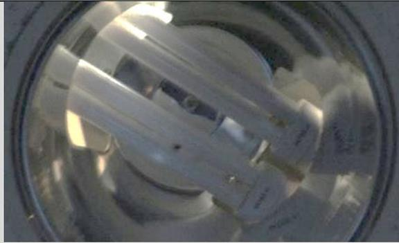
A recessed can-type fitting with two CFL tubes.
