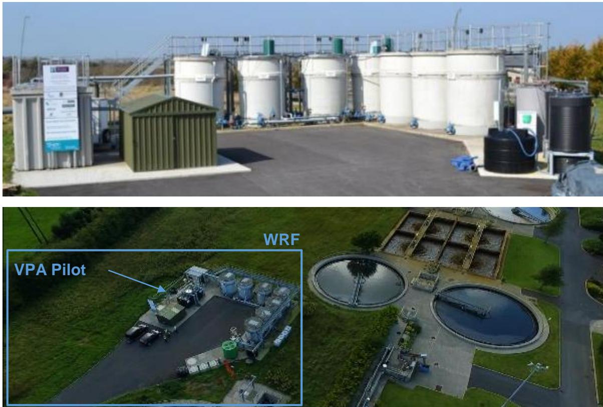
Figure 8: NUI Galway/ EPA Water Research Facility (WRF) Tuam WWTP, Galway, Ireland.
