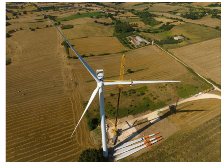
Figure 2 Re-blading of a Wind Turbine
