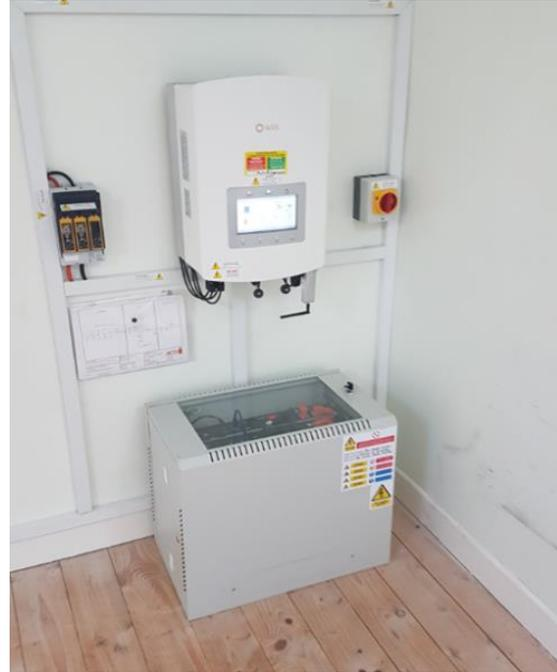
*Battery is installed in a suitable enclosure fixed in place on a fire-resistant surface or substrate (Class o) which extends 150mm beyond the edge of the system.*
