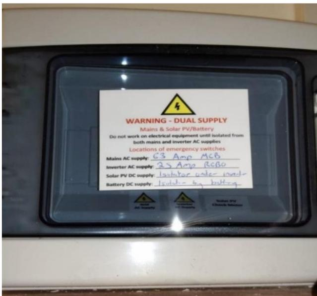
Fuseboard has dual supply warning label with emergency switches clearly labelled. Dual supply and emergency switches label must be present on all distribution boards.
