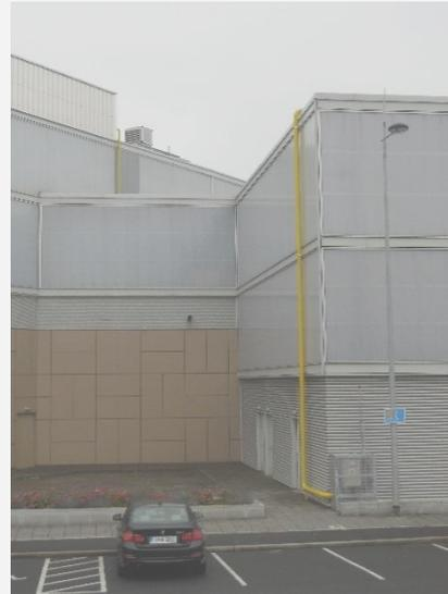
Figure 26: Gas piping to roof-mounted units in phase 2
