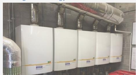
Figure 36: Wall-hung Gas Boilers 5x 100kW
