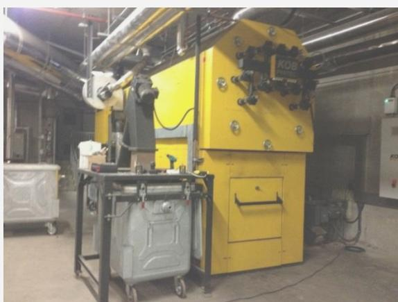
Figure 29: KOB 1.2 MW wood pellet boiler (photo Kaizenenergy.ie)
