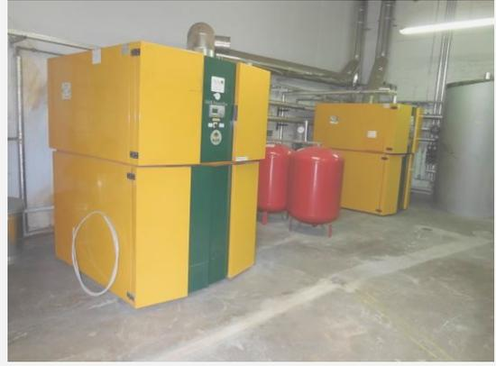
Figure 39: Wood pellet boilers in energy centre
