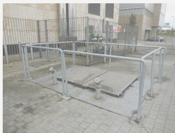
Figure 30: Ground level fill point for wood pellet store
