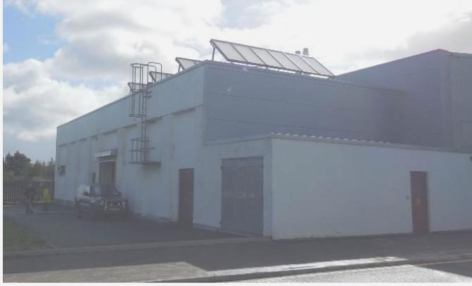
Figure 38: Existing Energy Centre with rooftop solar thermal
