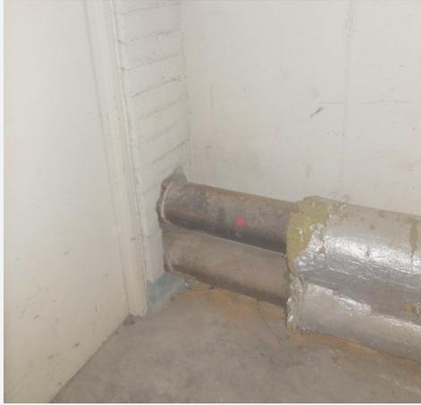
Figure 31: No insulation through brick wall
