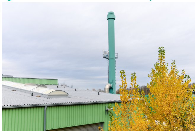
Figure 7.1: Stack from an odour treatment plant
