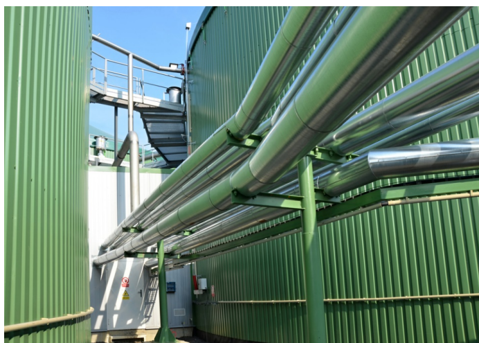
Figure 7.2: Biogas pipework and anaerobic digester tanks
