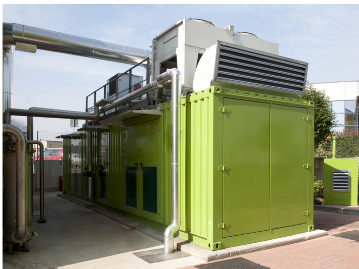
Figure 2.1: Typical containerised gas engine
