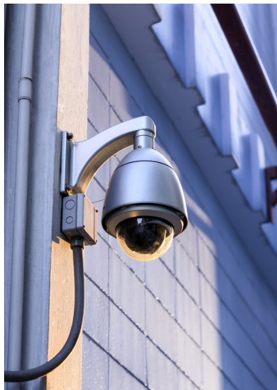
Figure 2.2: Typical pan/tilt/zoom closed-circuit television camera
