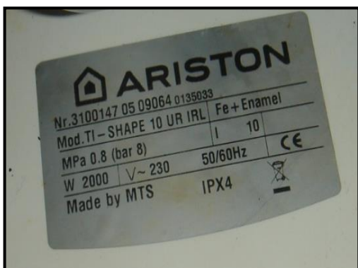
Figure 8.25: Instantaneous water heater data plate
