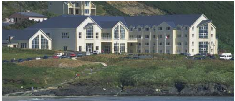
Inchydoney Island Lodge and Spa, Co. Cork plan to install a 500kW wood pellet boiler in 2005. This will be the largest wood-fuelled space heating installation in Ireland to date.
