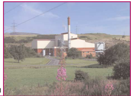
Poultry-fired combustion plant at Fife, Scotland
